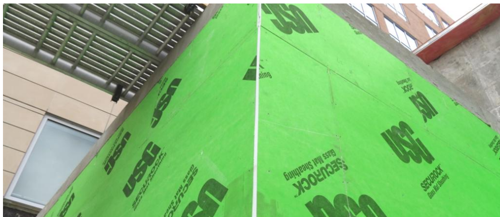
Nice Installation of the sheathing corner
